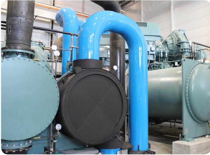
A **chilled water system**, also known as a “chilled water air-conditioning system,” employs water chillers to remove heat from liquids via a vapor compression or absorption refrigeration cycle. Once cooled, the liquid flows through pipes in buildings and passes through coils in air handlers, fan coil units, or other systems to cool building air.
