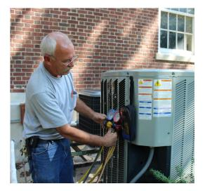
PROFESSIONALS IN THE PIPE TRADES BUILD AND REPAIR ALL OF THE COMPLEX SYSTEMS THAT RELY ON THE CIRCULATION OF LIQUID, STEAM OR GAS. THREE SHOPS FALL UNDER THE PIPE TRADES CATEGORY: REFRIGERATION, PLUMBERS, AND PIPEFITTERS. EACH SHOP RUNS TWO CREWS; ONE ASSIGNED TO MAINTENANCE ZONES AND ONE ASSIGNED TO CONSTRUCTION SERVICES.
